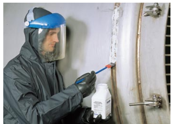
Avesta Classic Pickling Paste 101 – for brush pickling in all positions.
