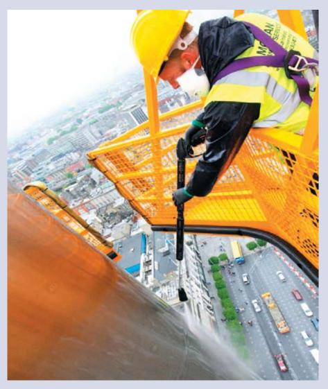
is suitable for pickling large surfaces, such as when the removal of iron contamination is also required.
